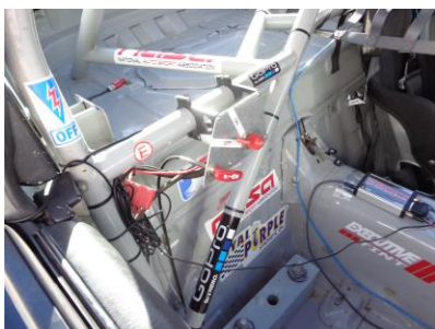
Little decal may cause confusion as fire handle is between electrical cut off symbol and electrical cut off switch.
